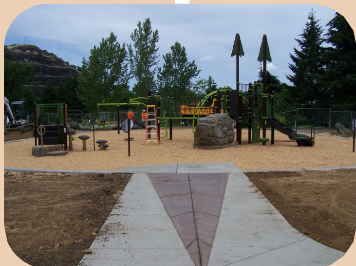
New playground almost completed
