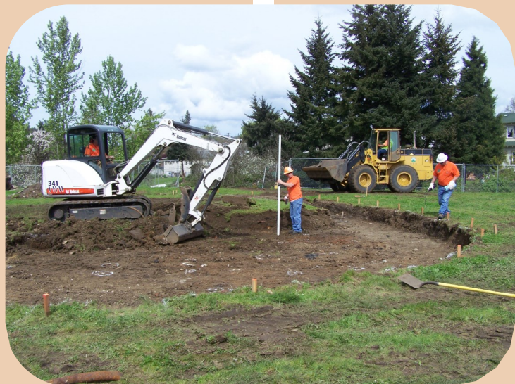
Excavation begins for the new playground
