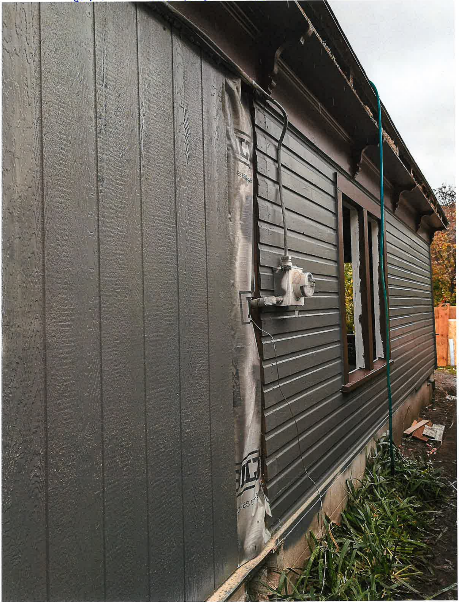
(E) PICS: NORTH SIDE WALL @ ENCLOSED PORCH
