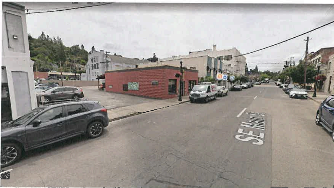
The above image shows the project site, as seen from SE Main St.
