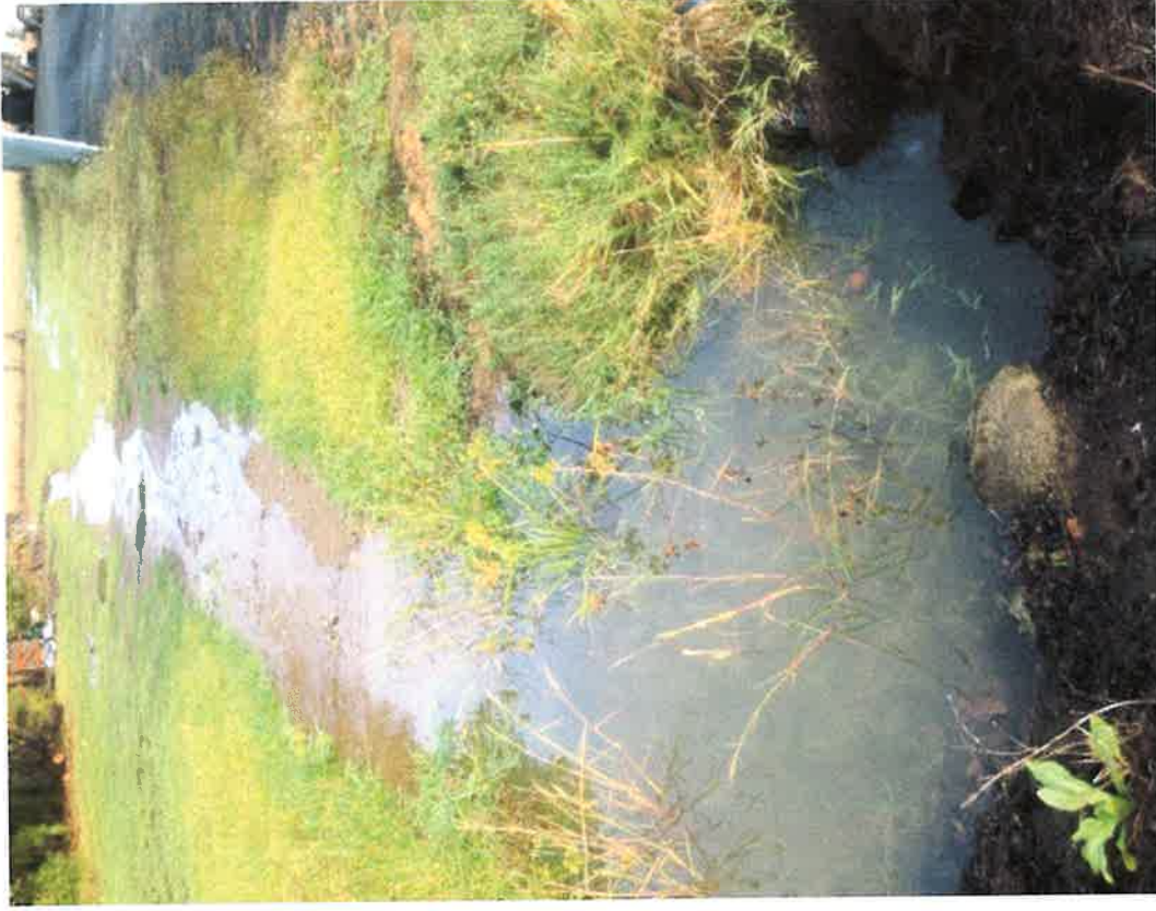
Looking north from Troost. Note culvert under road.
